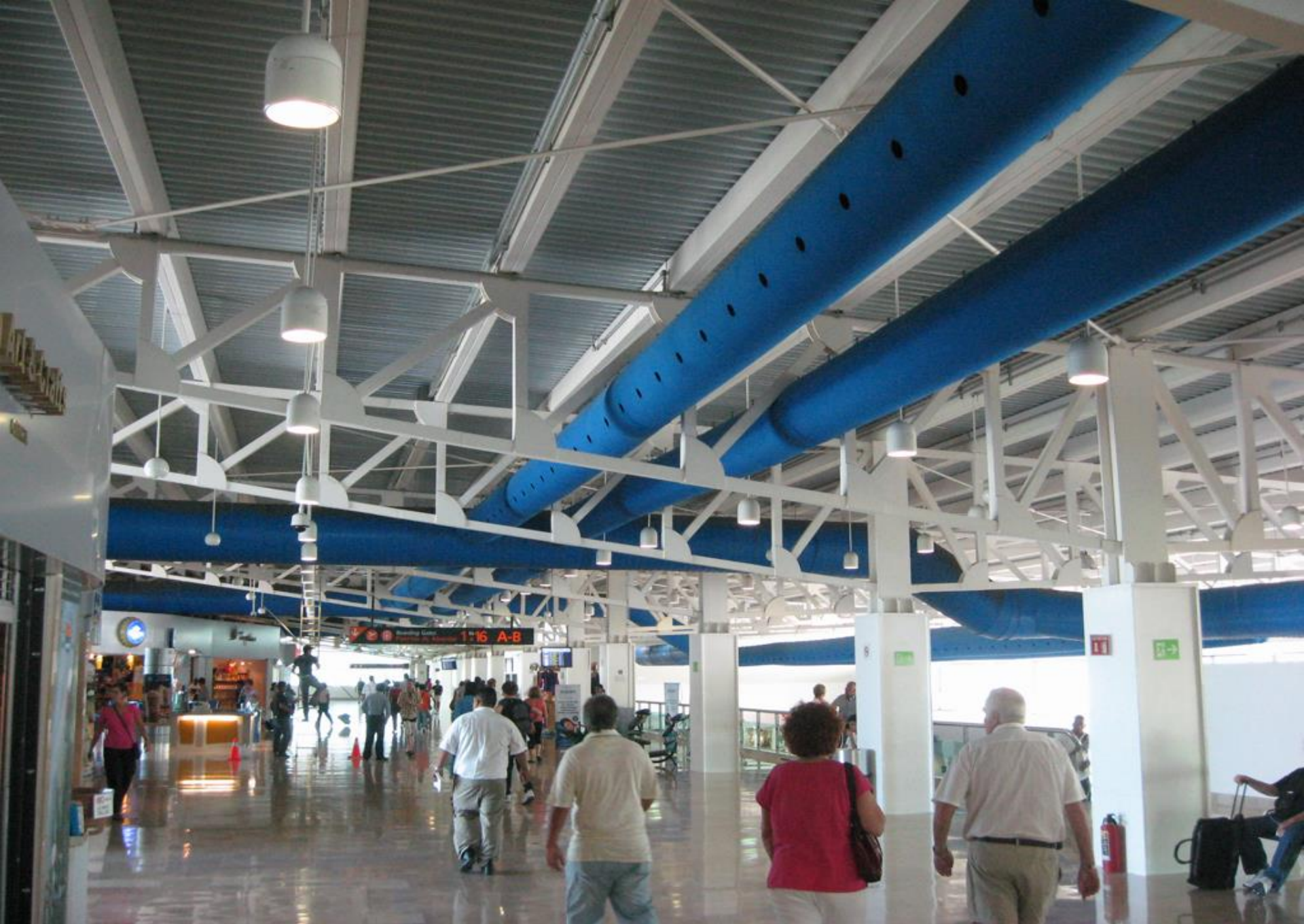
Puerto Vallarta Airport Terminal-Puerto Vallarta, Mexico
