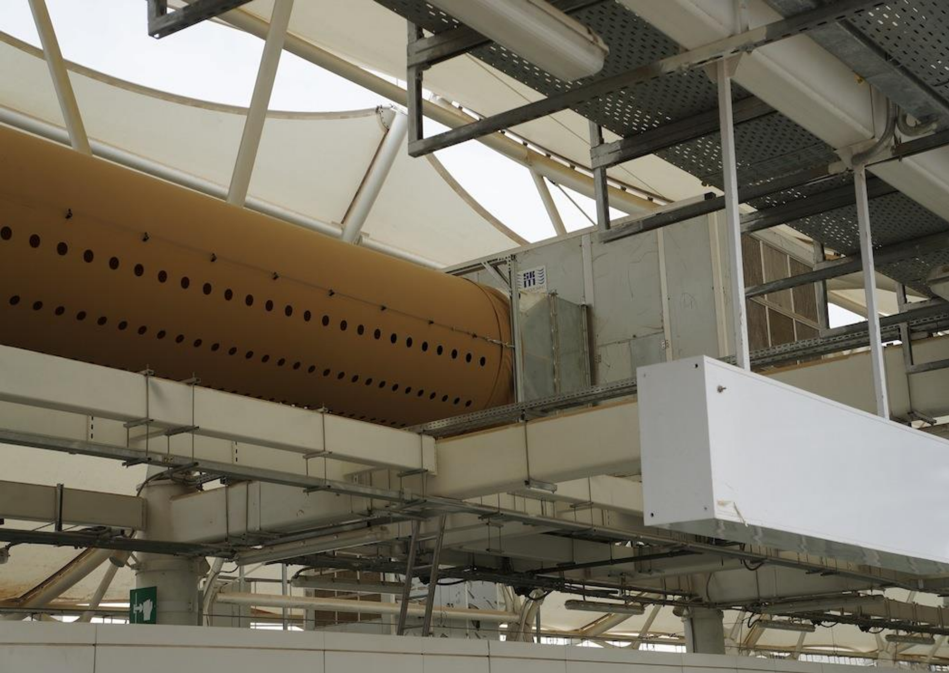
Mekkah Train Station-Mekkah, Saudi Arabia
