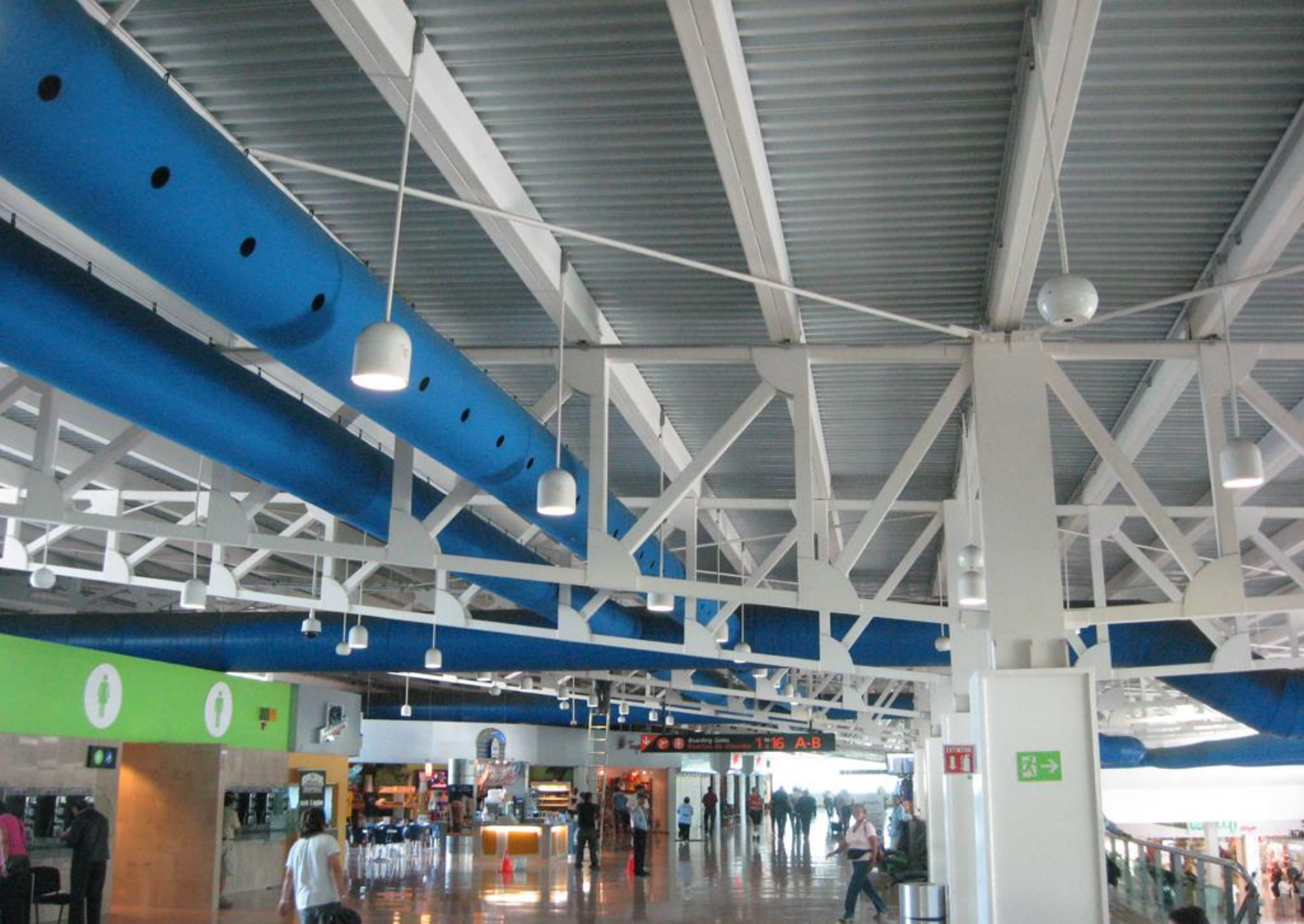
Puerto Vallarta Airport Terminal-Puerto Vallarta, Mexico
